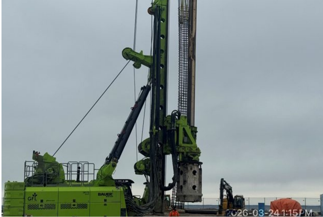
Structural caisson installation for new Membrane Filtration building
