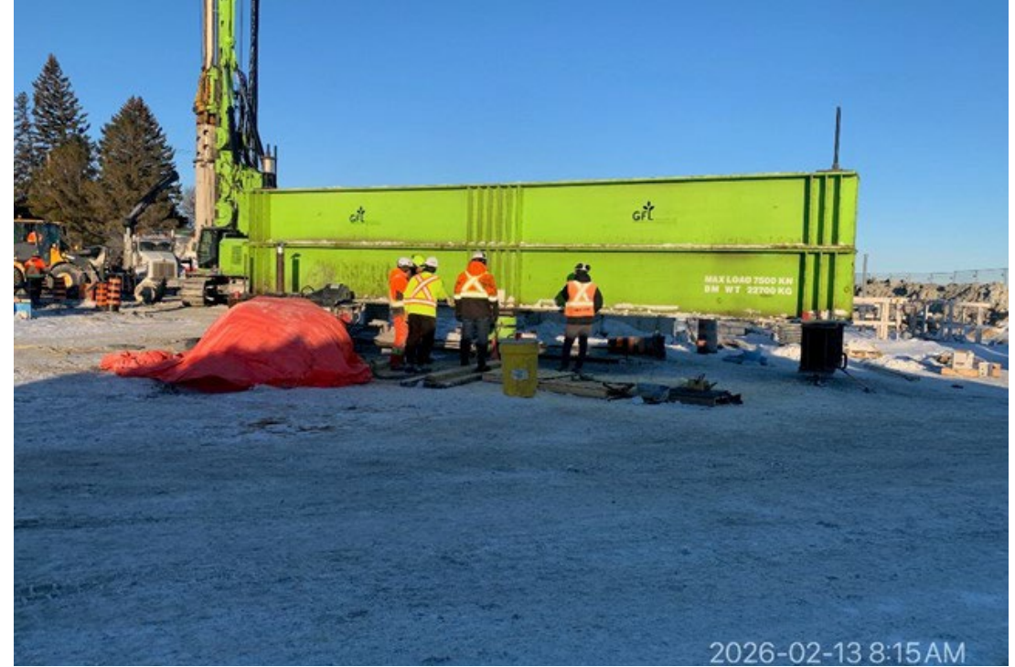
Structural caisson compression load test in progress.
