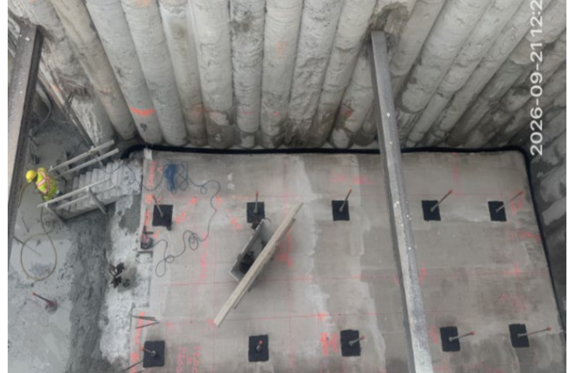
Foundation Layout on Poured Concrete Working Slab in Membrane Building Excavation
