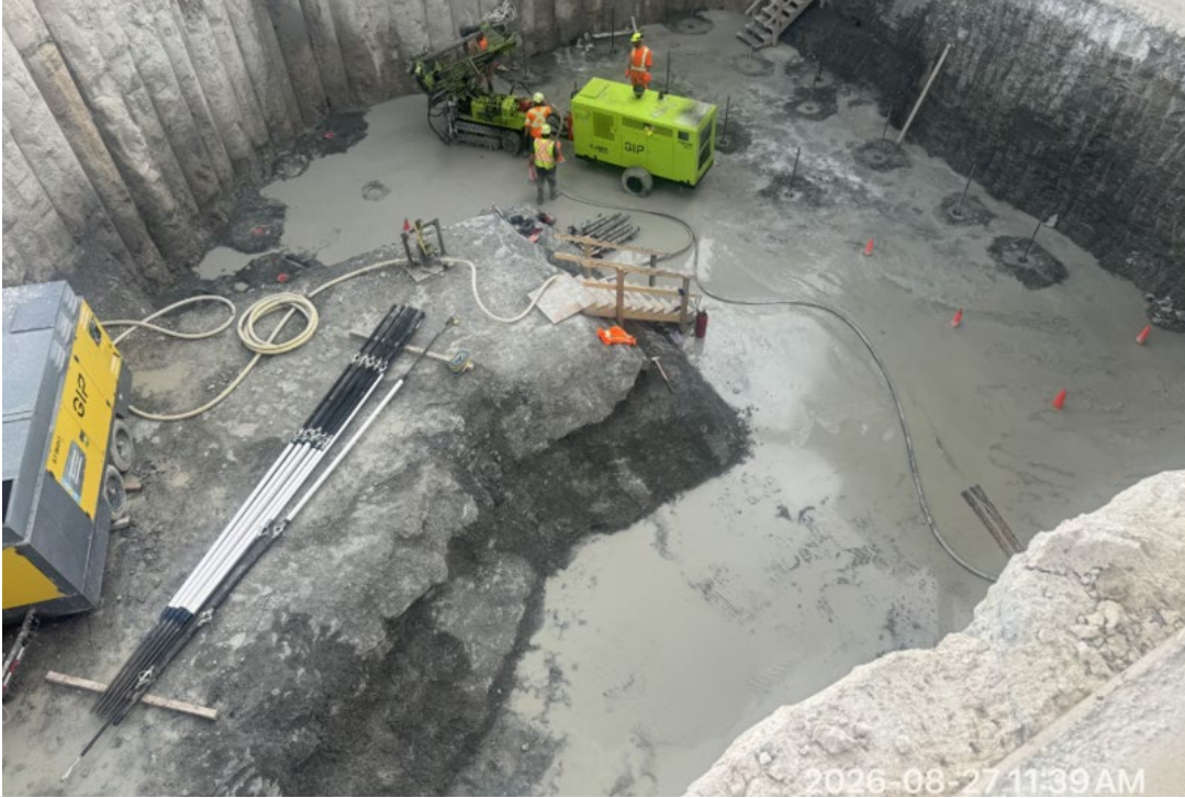
Rock Anchor Installation in Membrane Building Excavation
