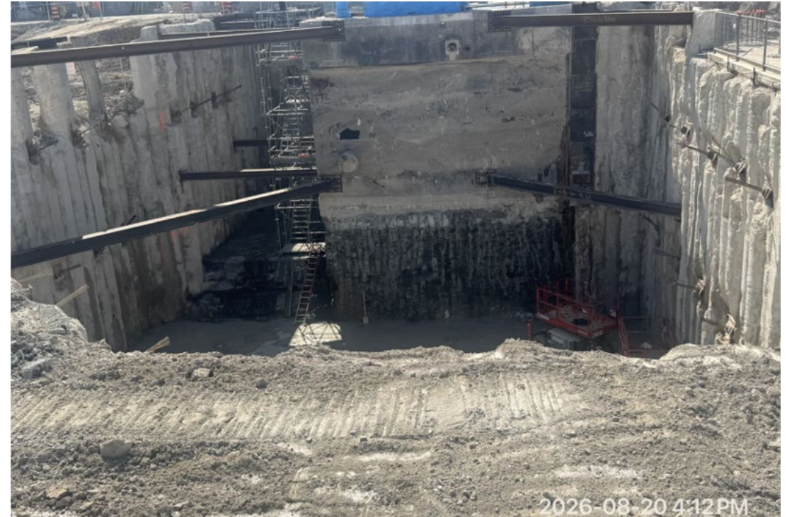
New Membrane Building excavation to Lower-Level. Temporary Bracing to Existing Raw Water Chamber for Lateral Support
