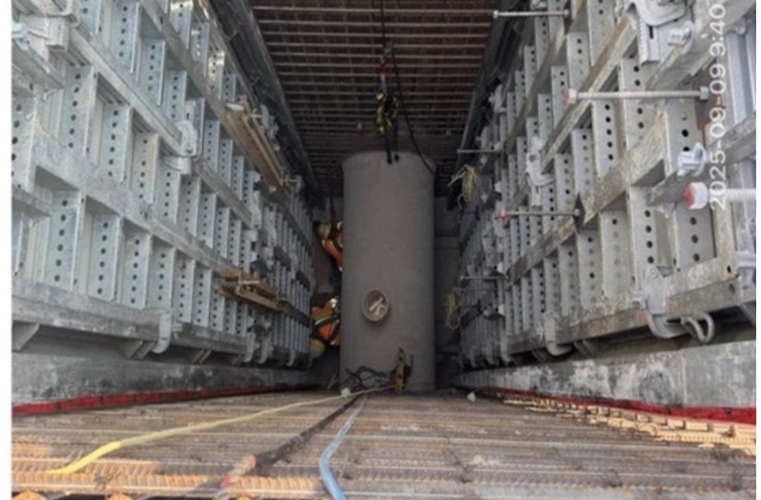
Installation of rebar and formwork for the walls of Intake No. 1 Chamber
