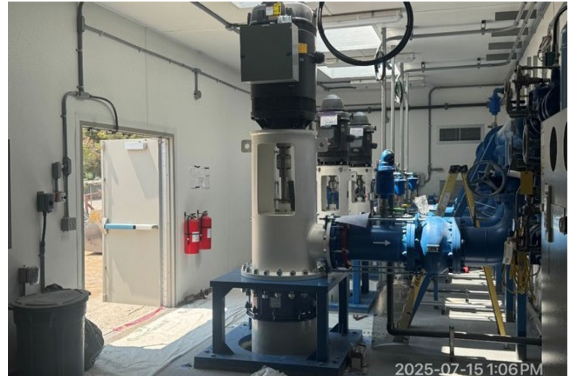
Installation of equipment (pumps, piping, valves, electrical, mechanical) within the temporary Industrial Pumping Station.
