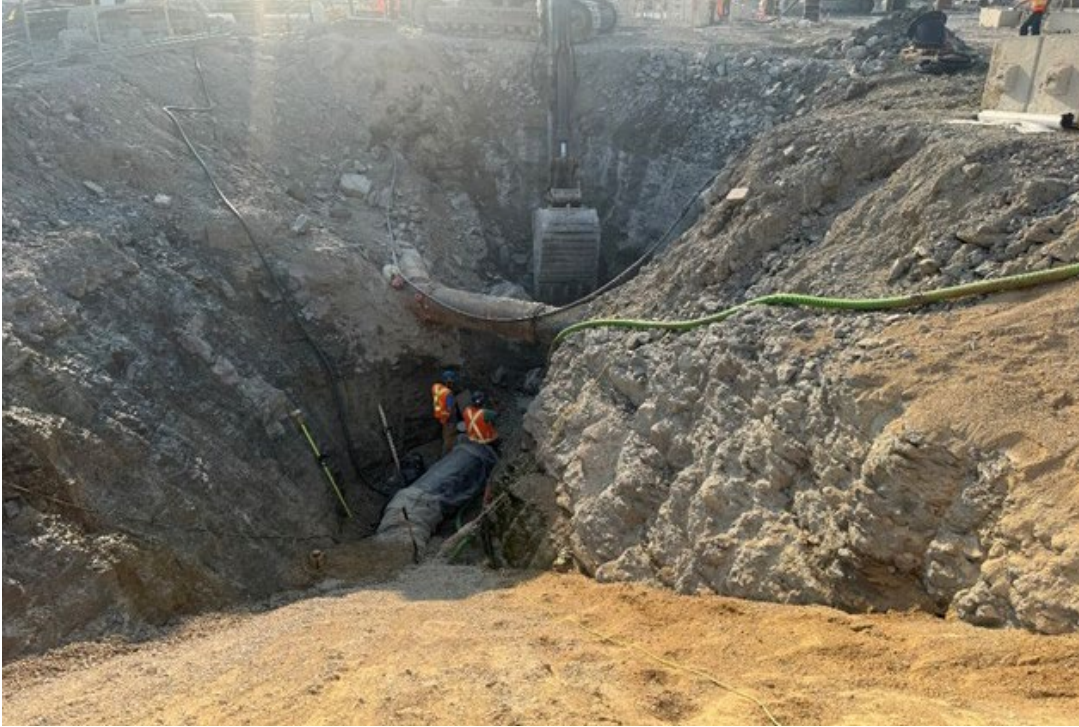
Installation of suction header piping between Intake No. 1 Chamber and the temporary Industrial Pumping Station.
