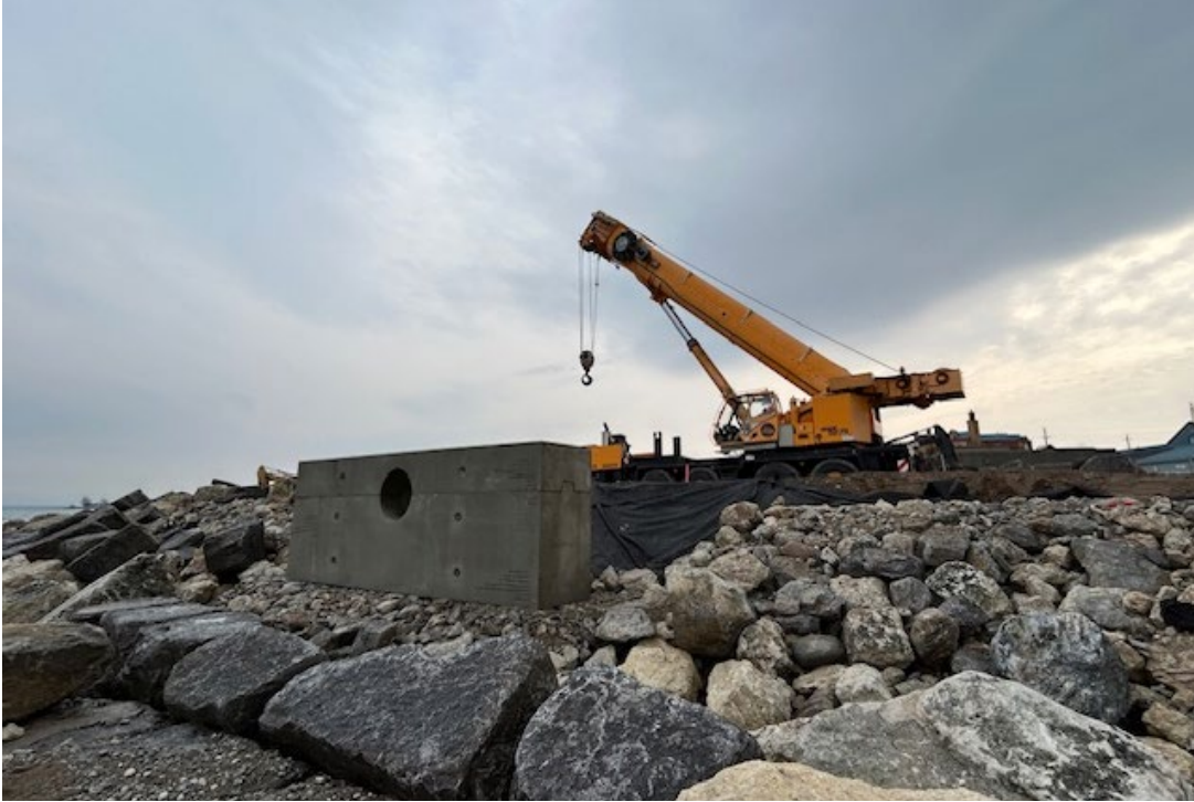
New headwall for future stormwater outlet.
