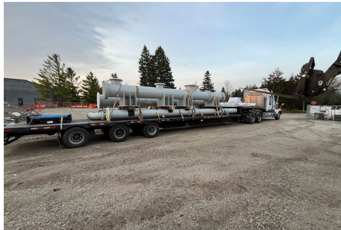
Process piping delivery for temporary Industrial Pump Station.
