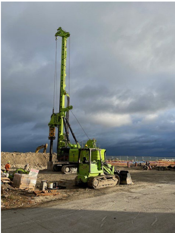
Drill rig installing caissons.
