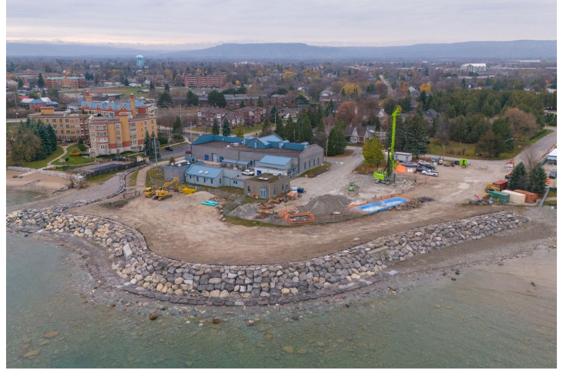
Shoreline reconstruction is complete.
