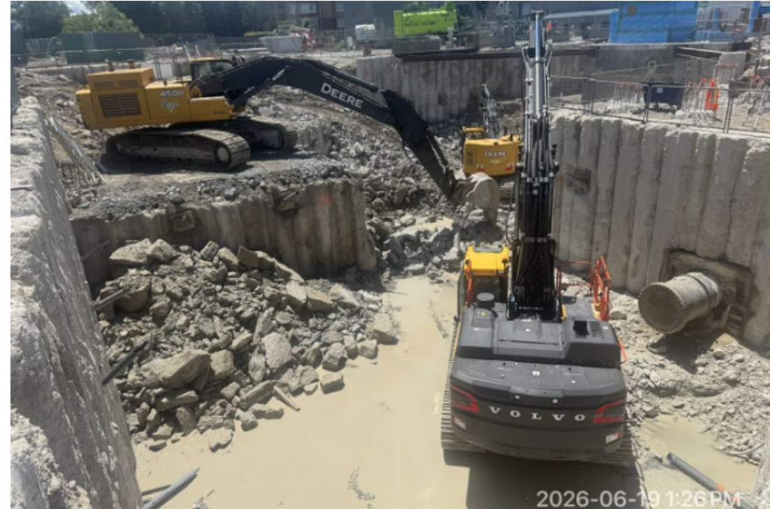
Deep Excavation for the New Membrane Building
