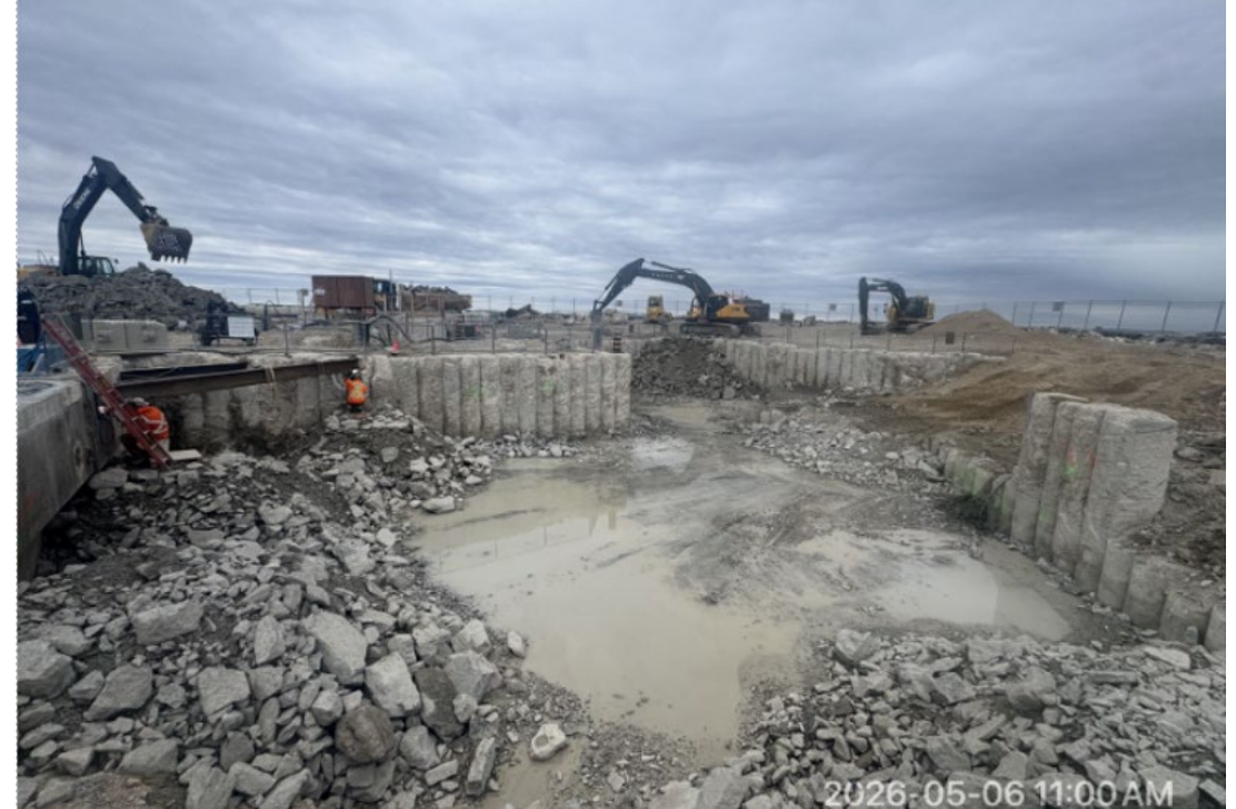
Excavation and rock removal for new Membrane Treatment Plant
