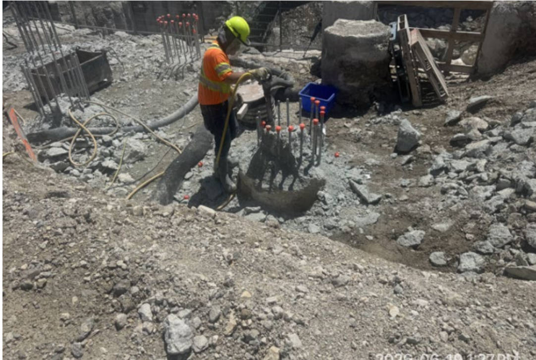
Preparing Concrete Structural Caissons for the new Membrane Building
