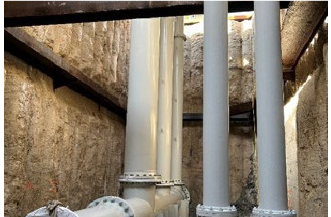
Pump suction columns and surge relief pipes installed in temporary Industrial Pumping Station excavation.
