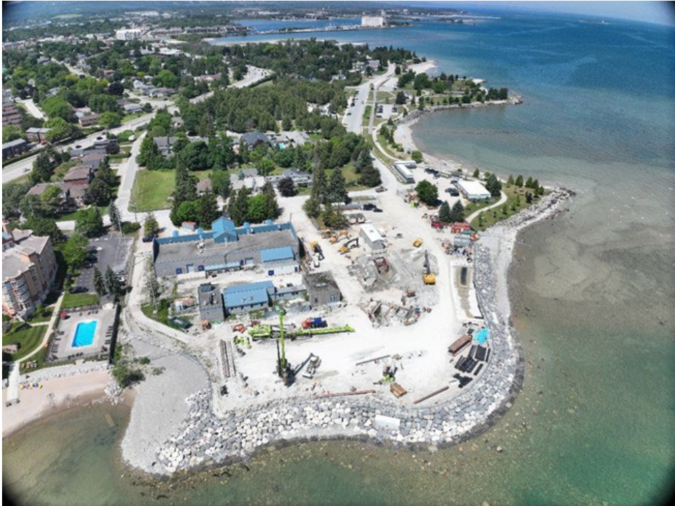
Site aerial photo June 2025. Construction dewatering area constructed in northwest corner.
