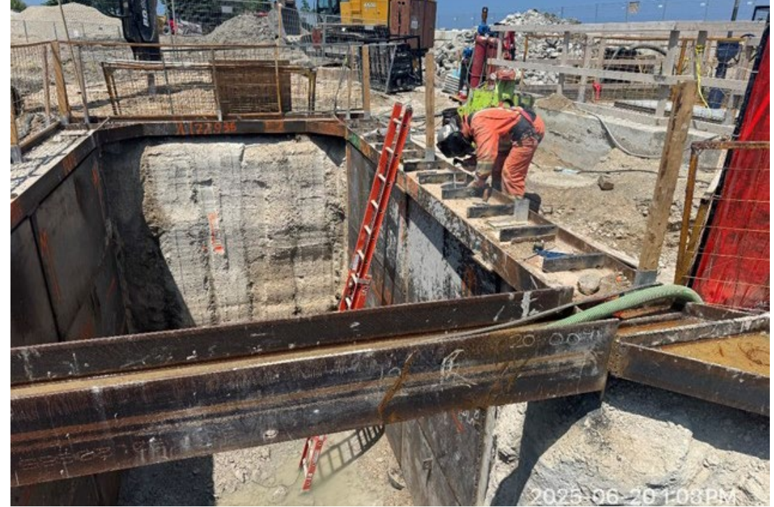
Excavation / Installation of Steel Plates / Installation of Waler at Intake Chamber
