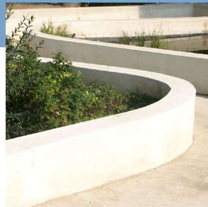
PLANTER WALLS: CAST-IN PLACE CONCRETE
