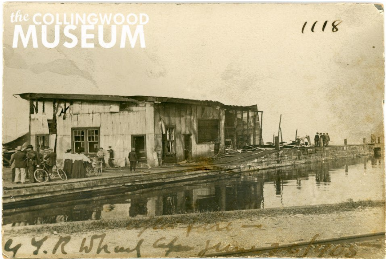
Figure 22 – Damage to the freight sheds from the 1905 fire (Source: Collingwood Museum, n.d. b)
